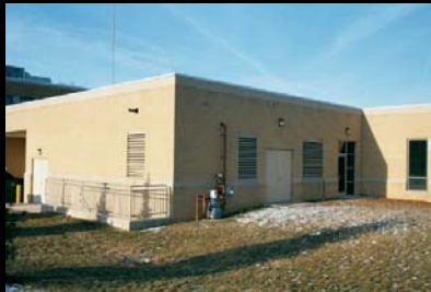
Circuits enter and leave the building under the snowy patch.
