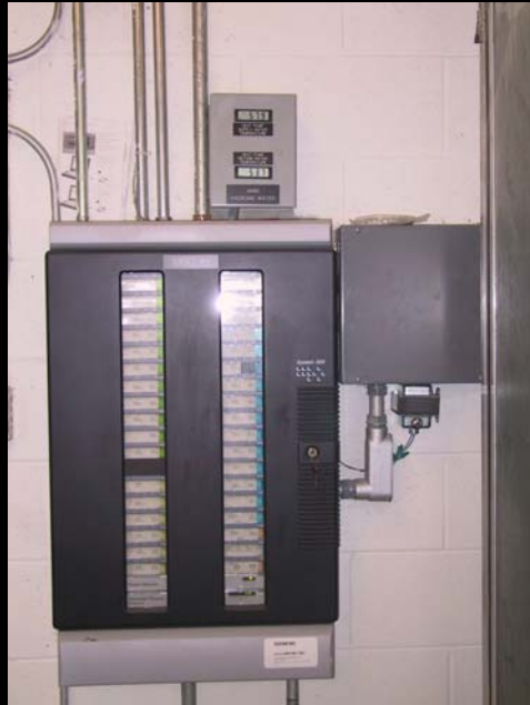
Central DDC controller and incoming / outgoing loop temperature meter
