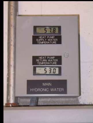
Central DDC controller and incoming / outgoing loop temperature meter
